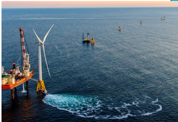
First wind turbines installed off shore US - August 2016
